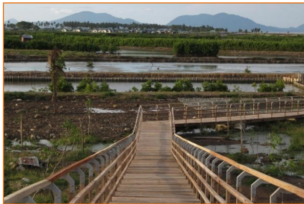
Picture 10. A view from Canopy Bridge facing the Weh Island
