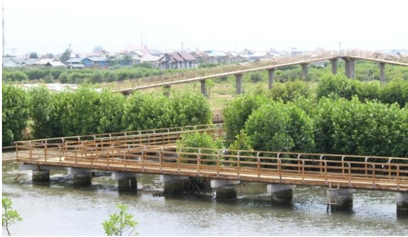
Picture 11. Bridge over the mangroves pond in Urban Forest
