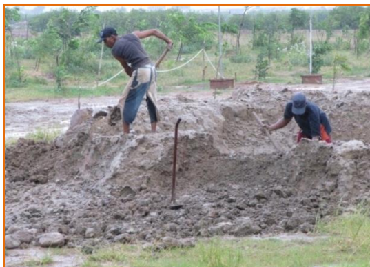
Picture 15. The construction of ponds
