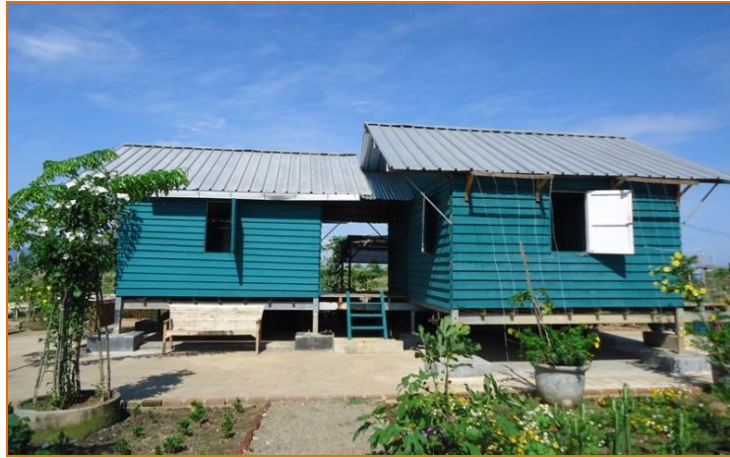
Figure 14: Shelter for City ForestBNI in Banda Aceh as a centre of activity and forest management
